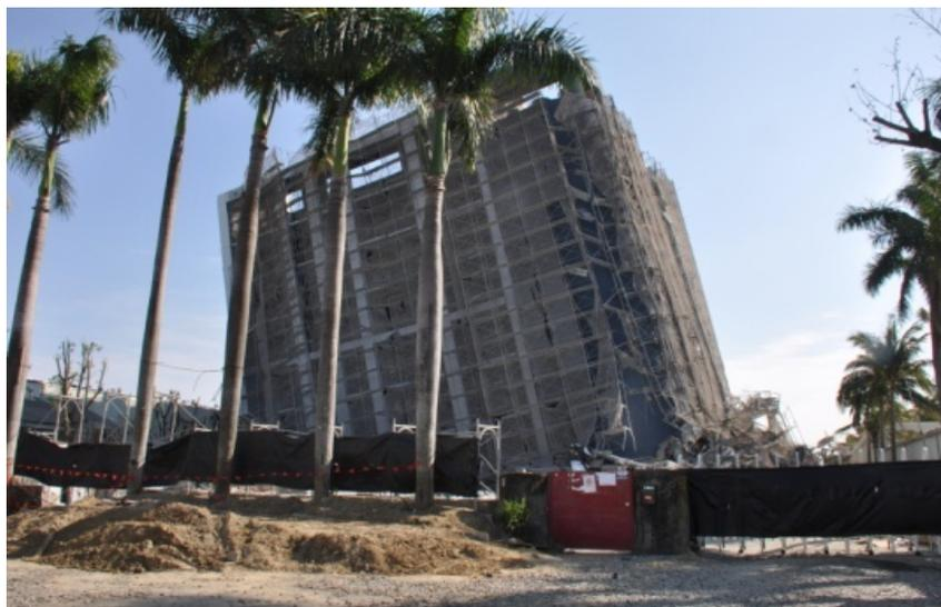
Figure 14. Tilting of a building induced by asymmetrical sliding failure of real foundation soil (Hsu and Ho, 2016).
